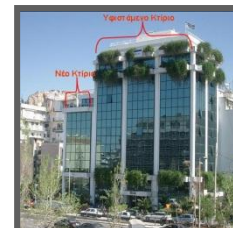
e-Management – energy buildings
