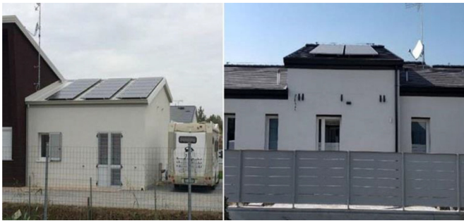
Fig. 3. PV panels on the rooftops of the residences.
