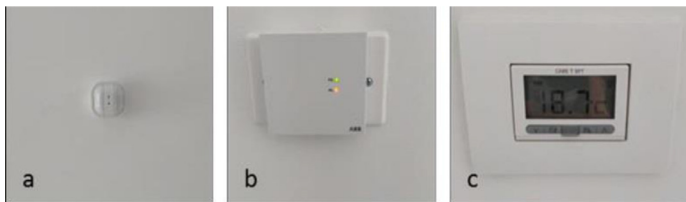
Fig. 6. a) Presence sensor, b) Air quality sensor, c) HVAC thermostat.
