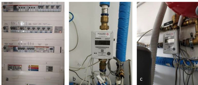
Fig. 7. a) Electricity metering, b) Heat pump energy meter, c) DHW meter.
