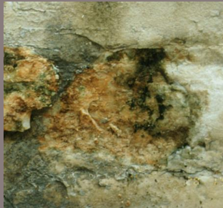
Stone's biodeterioration due to the development of microorganisms
